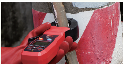
Measurement of Transformer Ground Resistance
