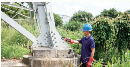
Measurement of Tower Ground Resistance
