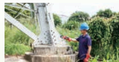
Measurement of Tower Ground Resistance
